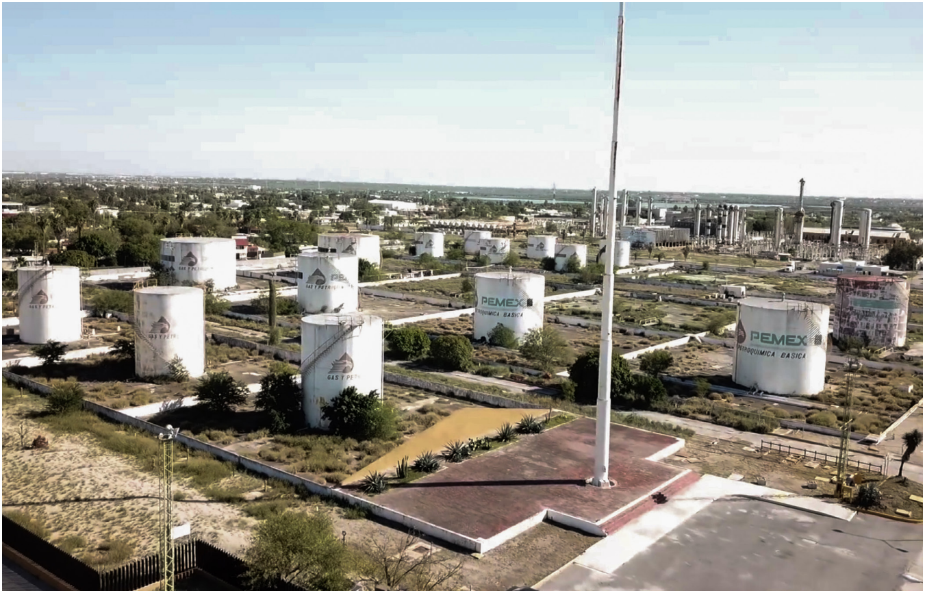
Figure 3. Existing Conditions. Image credit. Parque Refinería Reynosa Tamp.
